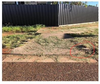
This damage was noted on 27<sup>th</sup> January 2023 where the pram ramp has been damaged due to Fencing work by Julalikari contractors. Location: Hilda and Blackmore st intersection
