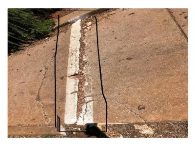
This damage was noted on  $14^{th}$  March 2023 due to LPOD pipes from IGA on our footpath causing damage and safety hazards. Location: Beside IGA (Pinnacles Rd).
