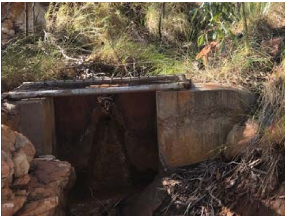
Photo 36 – Overview of the seepage weir.
