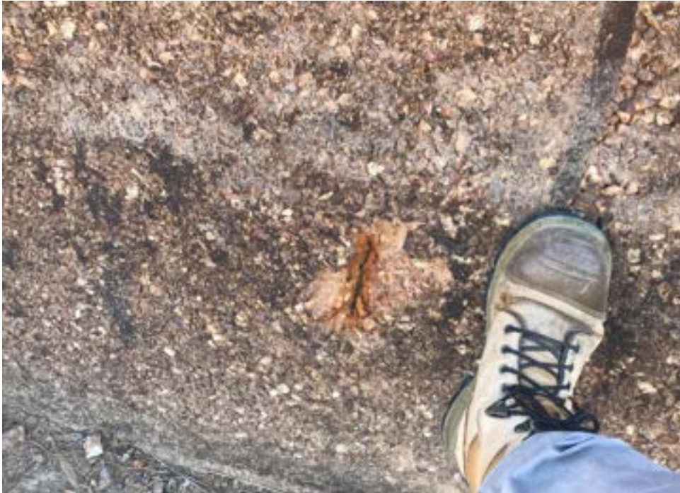
Photo 45 – Typical, spalled concrete on the upstream face of the spillway control weir.
