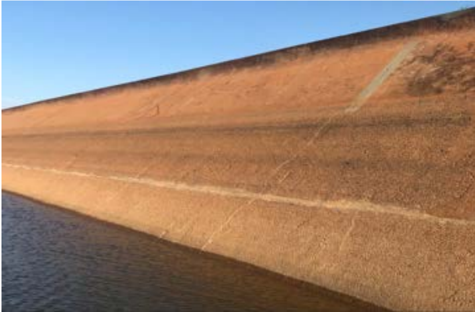
Photo 11 – Typical, cracking on the upstream face, viewed facing upstream. Joint repairs evident.
