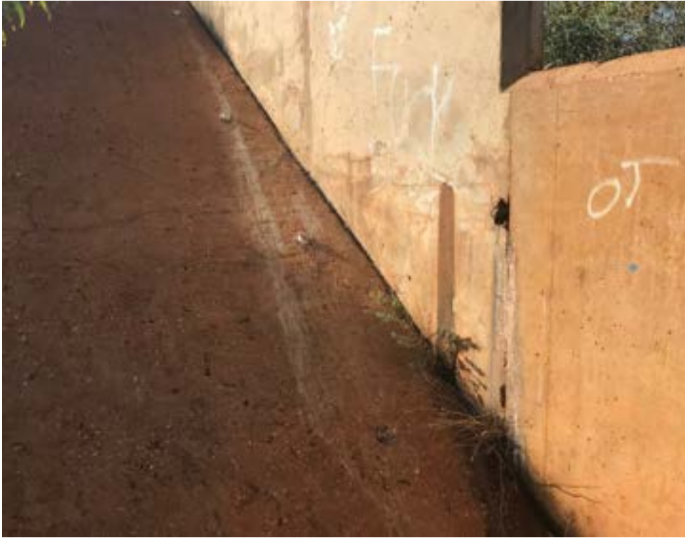
Photo 47 -Open and spalled joint on the downstream side of the spillway, right side.
