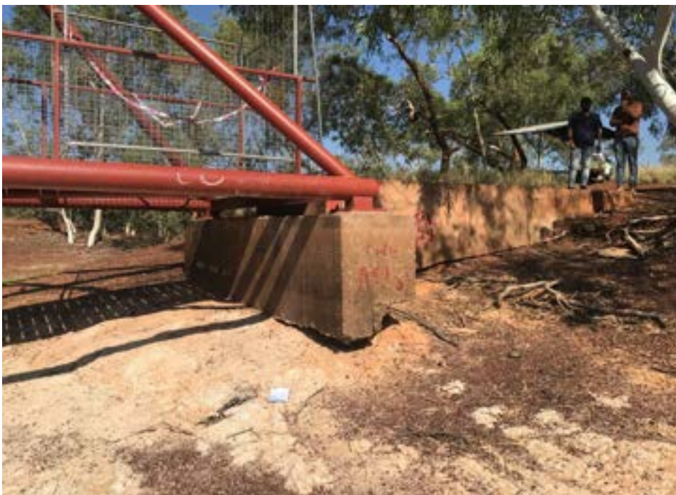
Photo 60 – Undermining of the pedestrian bridge abutment (2).
