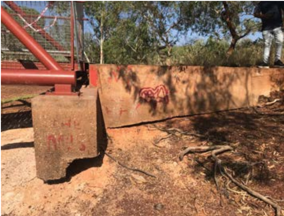
Photo 59 – Undermining of the pedestrian bridge abutment (1).
