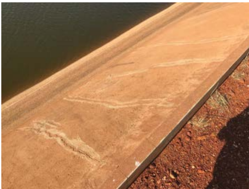
Photo 8 – Typical, cracking on the upstream face, viewed from the crest.
