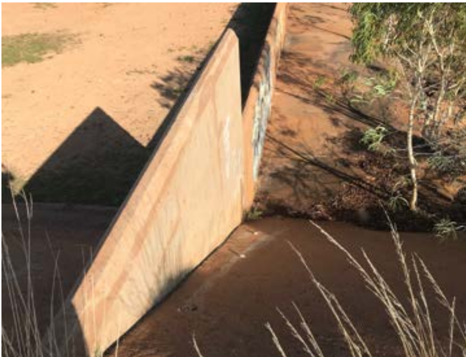
Photo 46 – Downstream apron and weir interface, right side.
