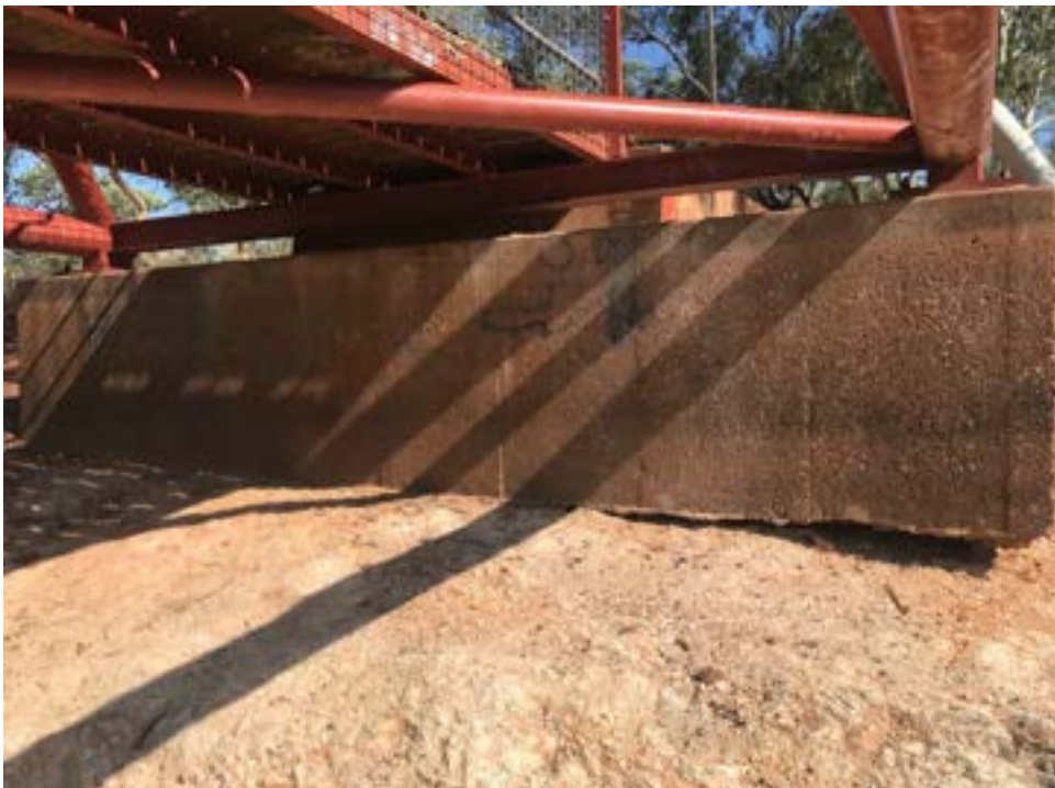
Photo 62 – Undermining of the pedestrian bridge abutment (4).
