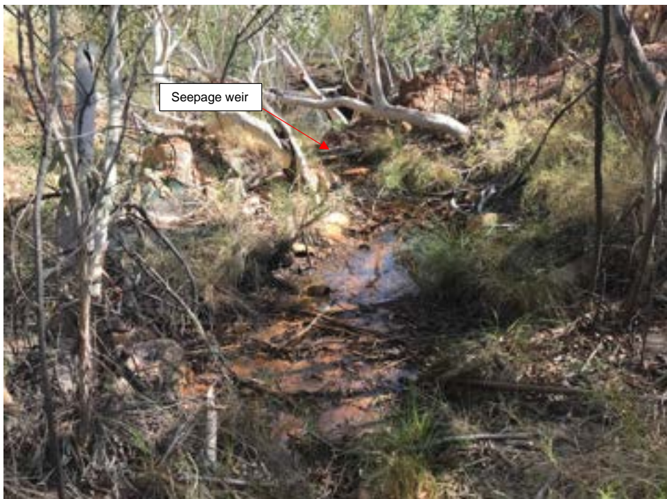
Photo 30 – Typical, seepage from the dam flowing toward the seepage weir (facing downstream).
