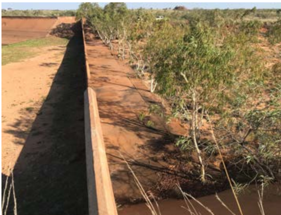
Photo 51 – Interface of the spillway apron and downstream unlined chute, facing left
