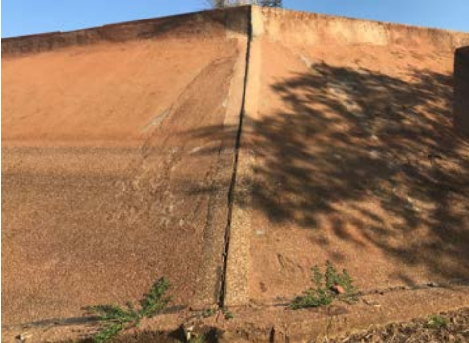
Photo 15 – Construction joint with filler at the right abutment.
