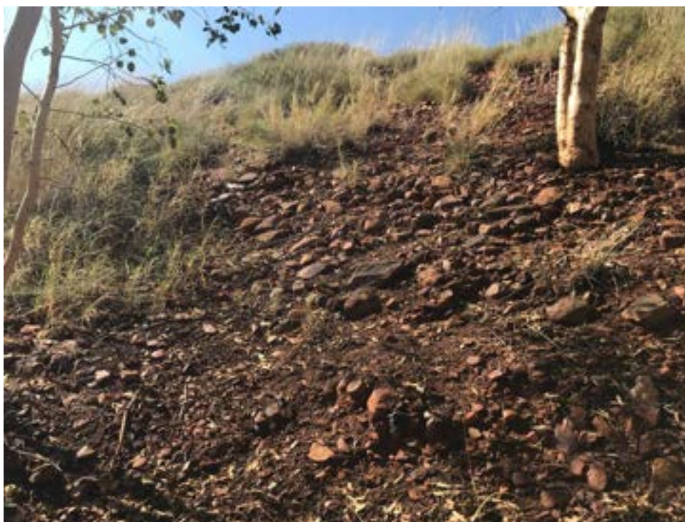
Photo 24 – Typical, exposed rockfill on the downstream face near the maximum section.
