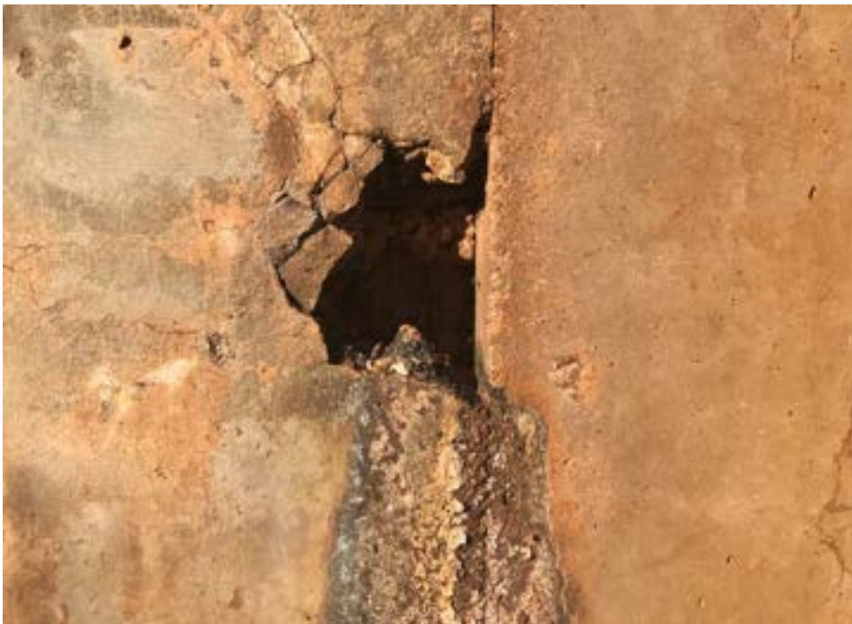
Photo 48 -Spalled joint as shown in Photo 47. Water stop could be seen in the joint.
