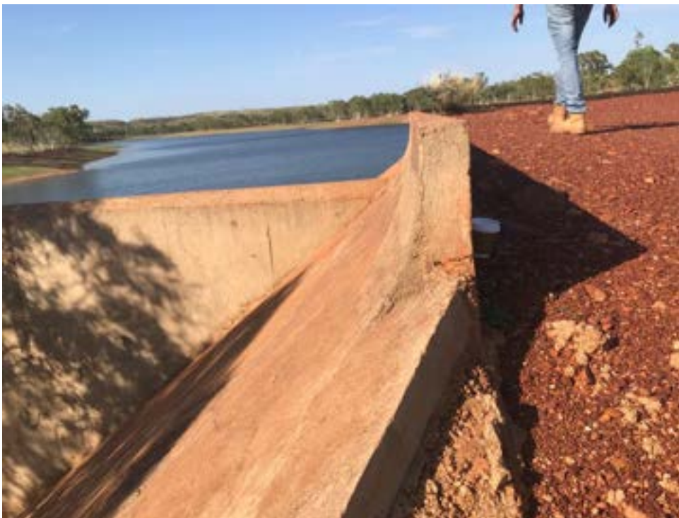
Photo 4 – Upstream face crest detail (wave wall).
