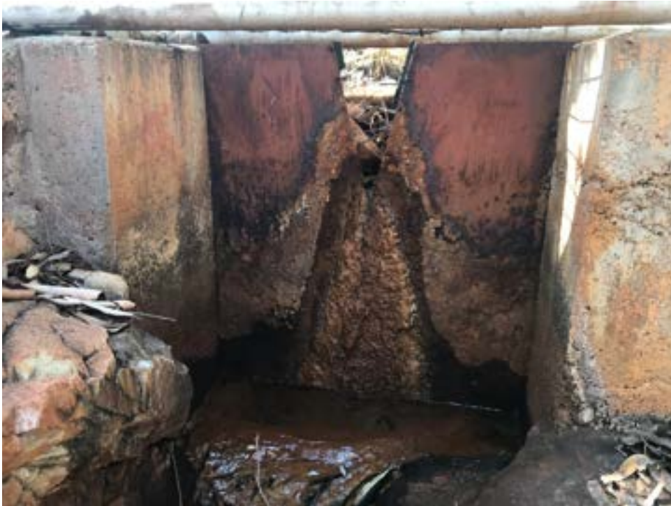
Photo 35 – Seepage weir current condition.
