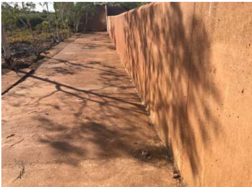
Photo 50 – Typical, concrete condition of the downstream side of the spillway and apron interface, facing right.
