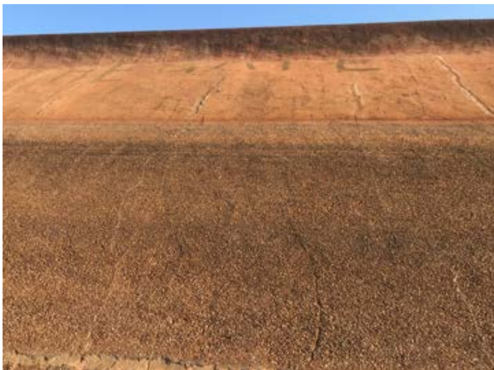
Photo 5 – Typical, cracking on the upstream face, viewed facing downstream from the boat.
