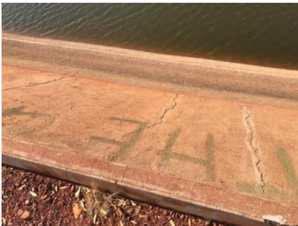
Photo 6 – Typical, cracking on the upstream face, viewed facing upstream.
