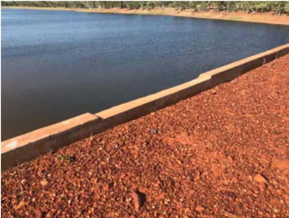
Photo 19 - Notch missing in the crest / wave wall.
