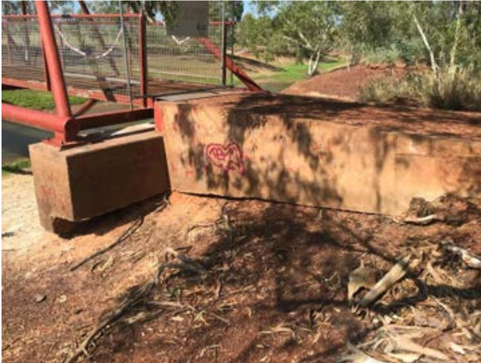
Photo 61 – Undermining of the pedestrian bridge abutment (3).
