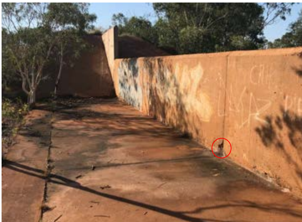
Photo 49 – Additional damaged joints on the downstream side of the spillway control weir, facing right.
