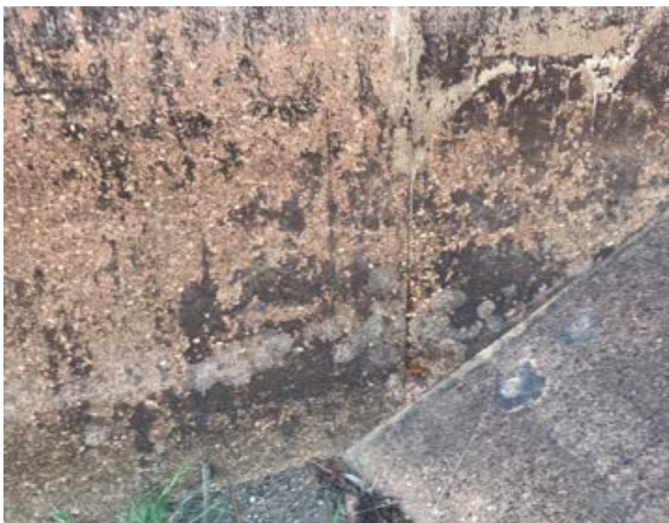
Photo 44 – Open joint on the upstream side of the spillway control weir, near the left abutment.
