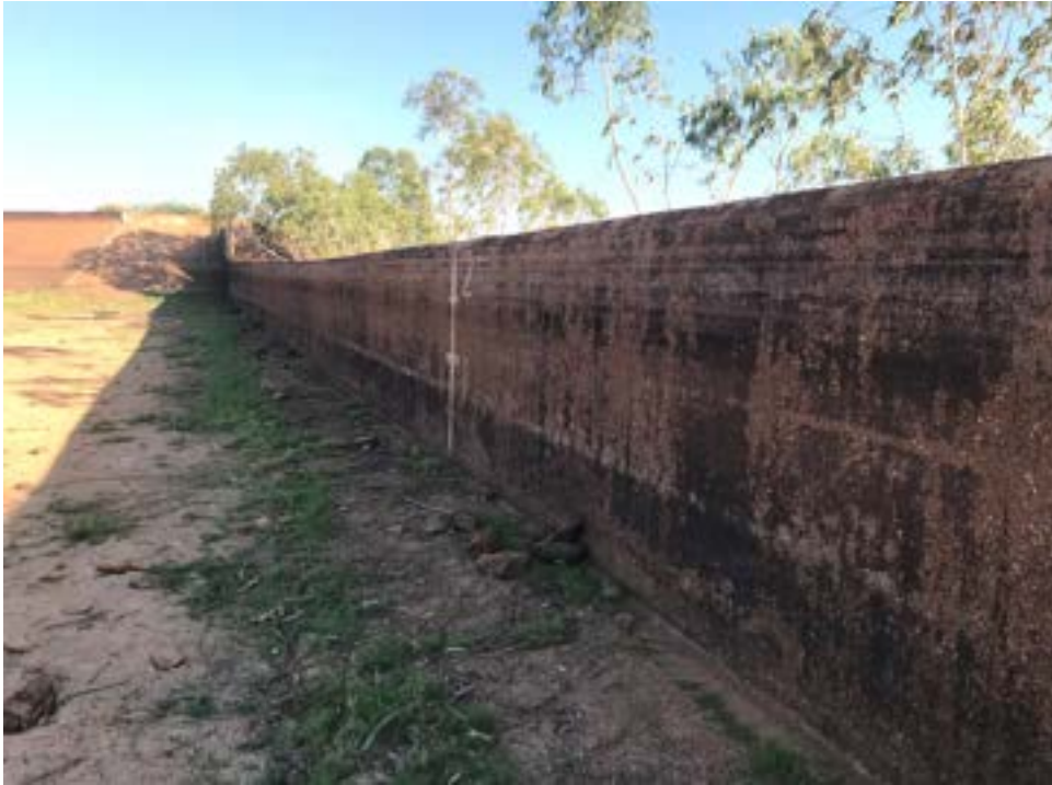
Photo 41 – Typical, upstream face of the spillway control weir.
