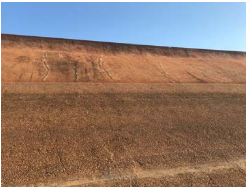
Photo 7 – Typical, cracking on the upstream face, viewed facing upstream. There is evidence of historical repairs being undertaken on the joints.
