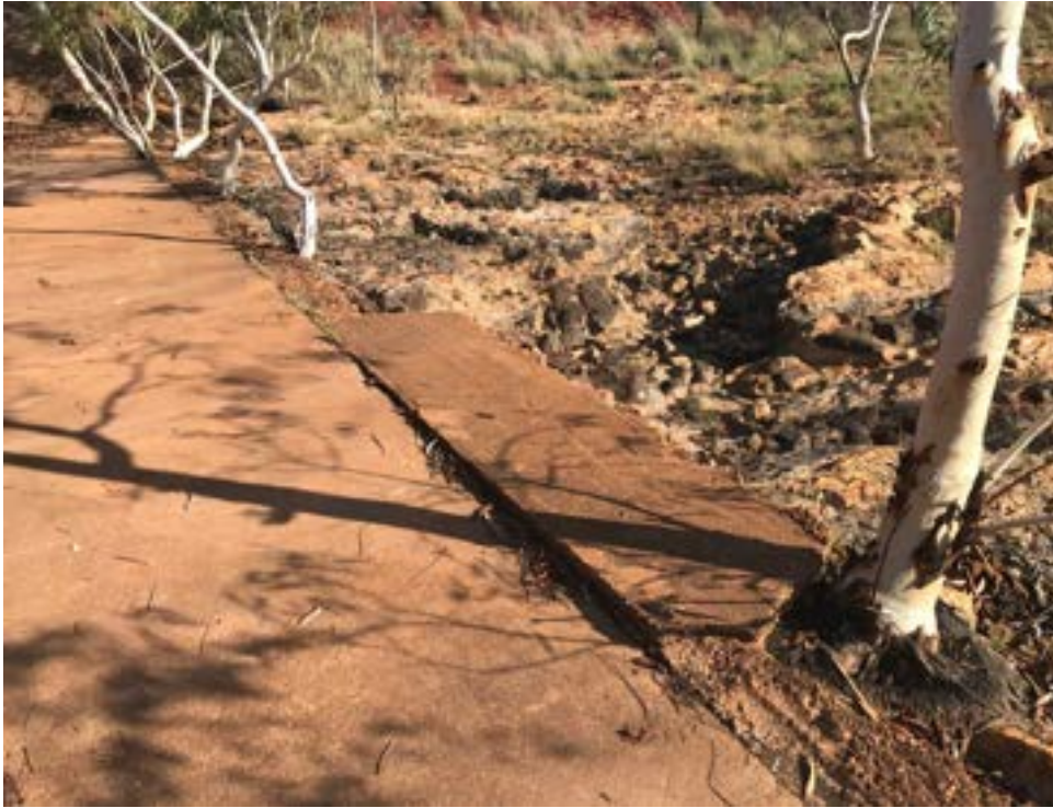
Photo 53 – Typical, sections of damaged concrete downstream of the apron, facing left.
