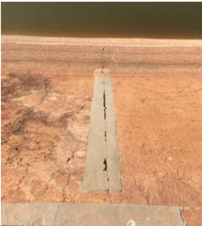
Photo 12 – Typical, cracking on the upstream face, viewed facing downstream. A repair attempt appears to have occurred.
