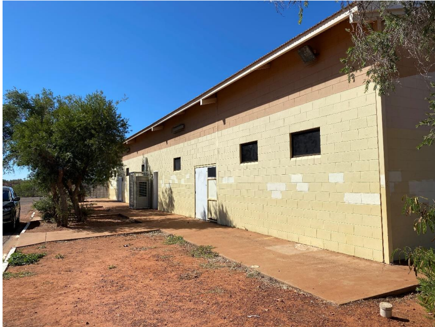
Figure 4 - External Paint Finish Showing Patch Work Repaint
